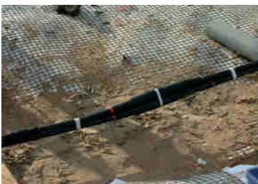
TS-24CSJ hybrid transition joint
