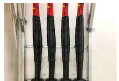
24CSJA-S cold-shrinkable straight joint
