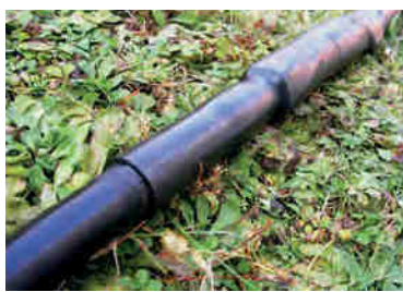
GTS1 heat-shrinkable straight joint
